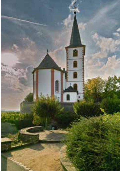
Church of St Peter and Paul in Hochheim
